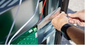
The inverters in the back have the DC output at the bottom of each slot, while the inverters in the front have the DC output at the top.
