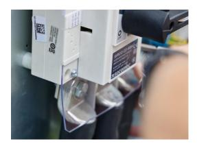
Connect the ground to the distribution block on the right of the EV Base Ultra, using an 8 mm hex wrench. Tighten it to **25 Nm**.
