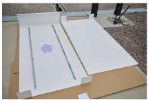
d. A top plate of the EV Base Ultra anchor is already mounted to the charging unit for easy installation. In order to place the EV Base Ultra on the installed anchor, first remove the dummy top plate of the installed anchor.
