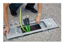
e. Place the EV Base Ultra (with floor plate) over the anchor. Make sure all holes align with sides of the anchor and the power supply and ethernet cables go through the central opening of the EV Base Ultra.
