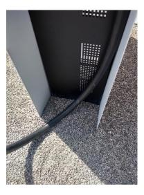
The EV Base Ultra can be placed maximum 3 cm below the top of the surrounding soil for aesthetic purposes. It cannot be placed lower as there will be risk of water ingress.
