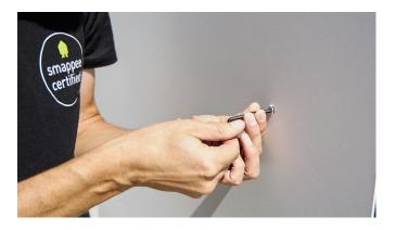
d. Use four screws to fix the top of the front plate, using a 5mm hex wrench. Front and back plate should align.
