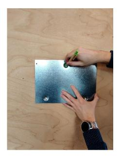
b. Drill 3 holes of 10 mm diameter through the slots to a depth of 50 mm. Insert the supplied wall plugs into the holes.
